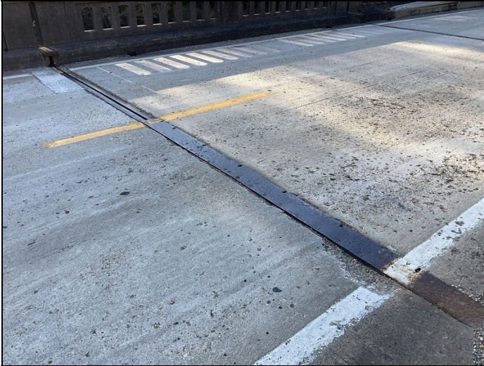
Joint - Bent 3: Sliding plate missing
