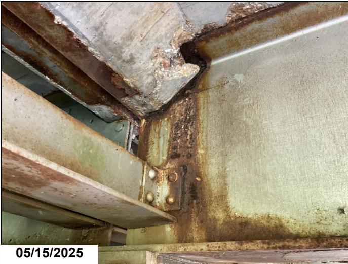
Span 3 Girder 2 left @ Bent 4: CS4 corrosion
