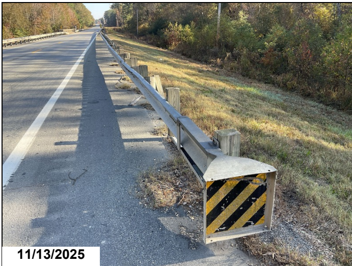
Approach railing - Bent 1 right: Post broken
