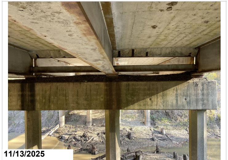
Cap - Bent 2: Debris build-up
