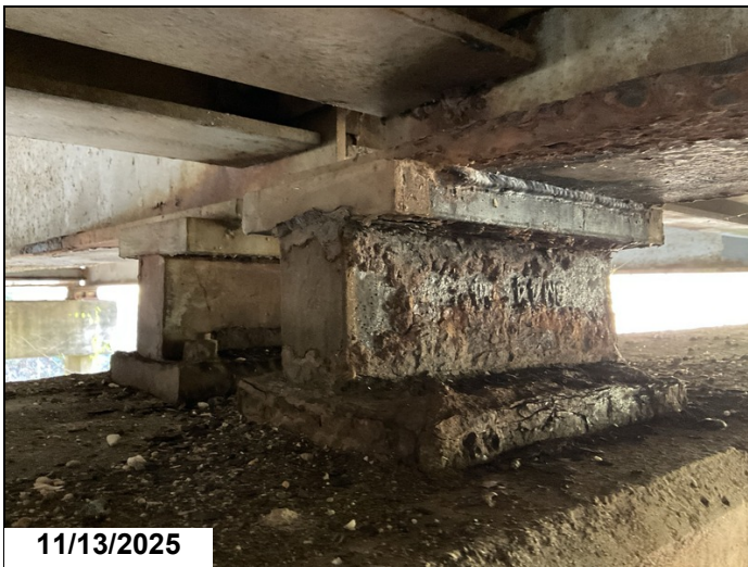
Bent 4 Bearing 2 ahead: Corrosion
