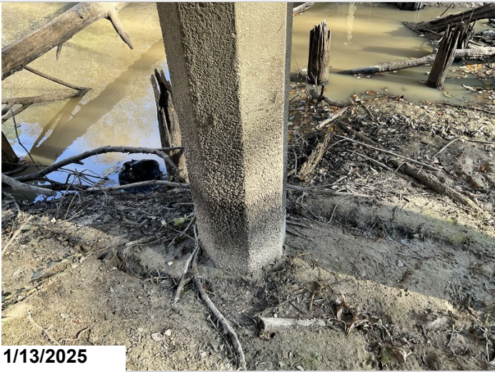
Bent 2 Pile 2: CS2 Abrasion/Wear
