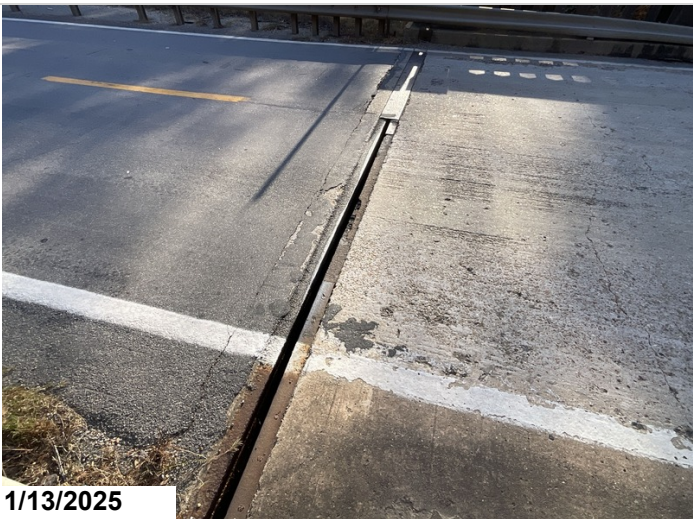
Joint - Bent 5: Sliding plate missing
