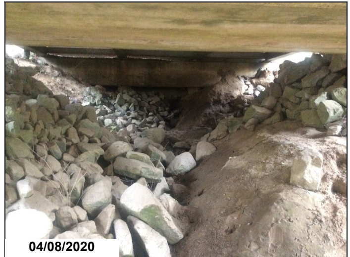
Endslope - Bent 5: Erosion
