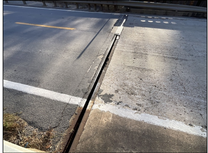
Joint - Bent 5: Sliding plate missing
