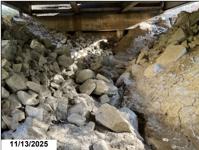
End-slope - Bent 5: Erosion
