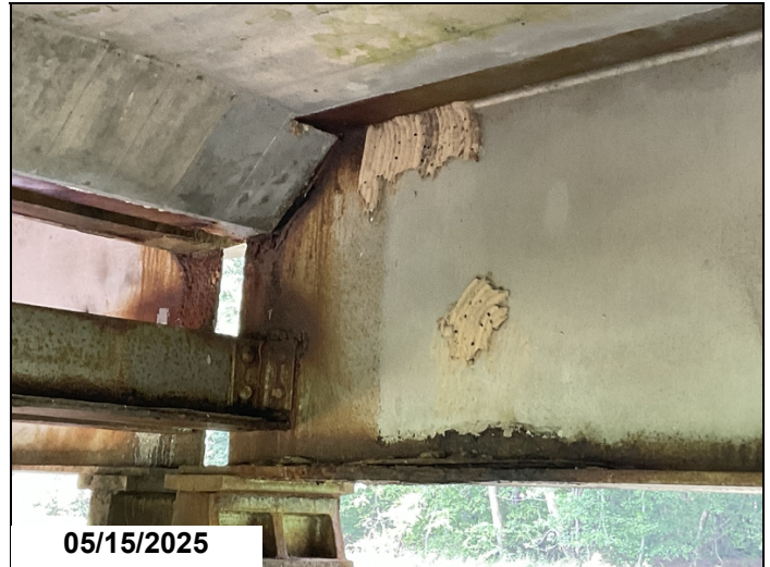
Spans 2-3 Girders 1 @ Bent 3: CS4 Corrosion
