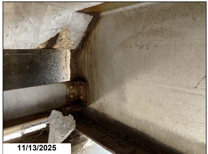
Span 4 Girder 4 left @ Bent 5: Corrosion
