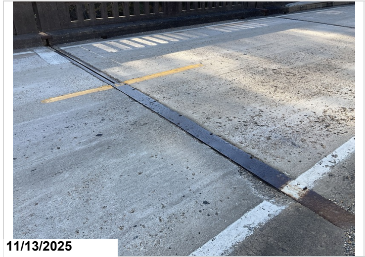
Joint - Bent 3: Sliding plate missing
