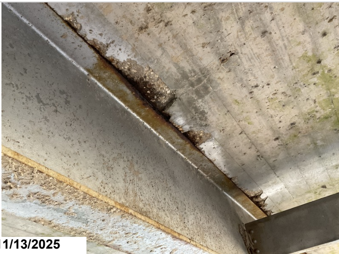
Span 3 Bay 2 @ Girder 3: Spall along edge of girder
