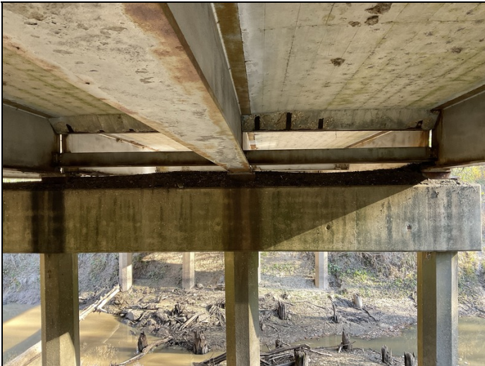
Cap - Bent 2: Debris build-up
