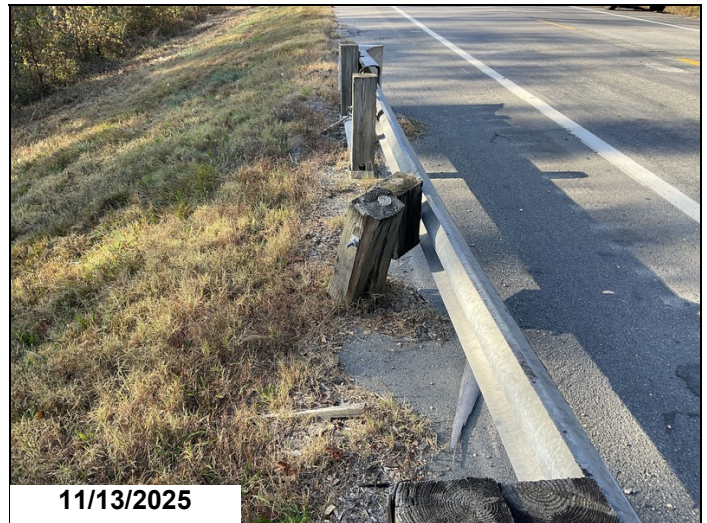
Approach railing - Bent 1 right: Damaged
